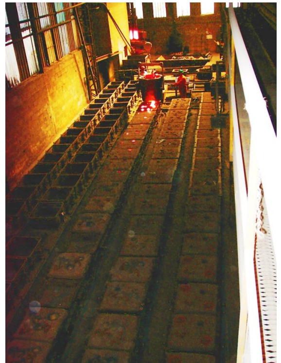
Semi automatic installation
